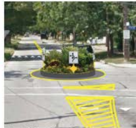
Traffic Circle (Cleveland)
